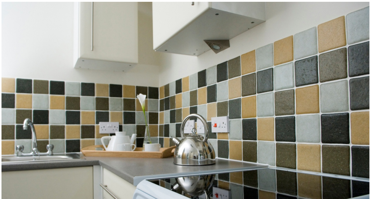
Figure 9, Recycled glass tiles installed in the kitchen
