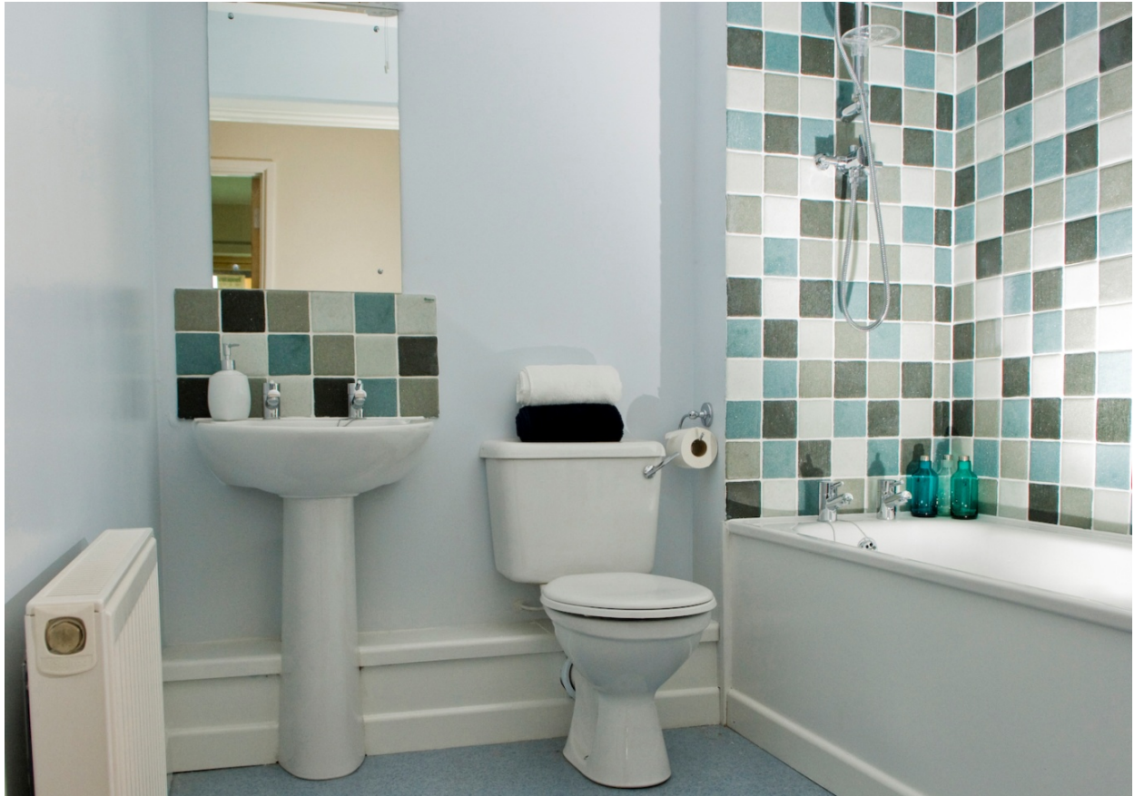
Figure 8, Recycled glass tiles installed in the bathroom
