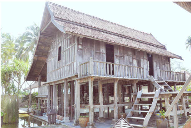
Figure 1: Example of a traditional Malay house in Terengganu with a regional variation of form and style influenced by Thai architecture. This structure was disassembled, reconstructed and restored as a resort building in Terrapuri heritage village.
