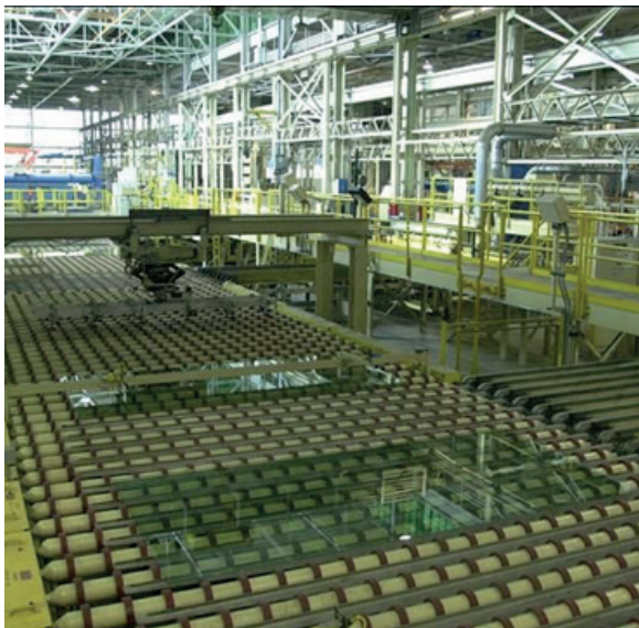
Burners over molten float glass.
